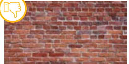
Brick wall to be insulated from exterior.
