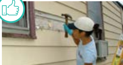
Insulation access holes plugged and sealed with solid plugs. Courtesy of U.S. Department of Energy
