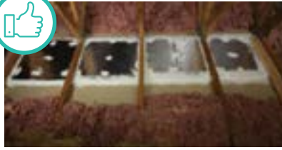
Sealed chase or cavity. Courtesy of Oregon Housing and Community Services and Oregon Energy Coordinators Association
