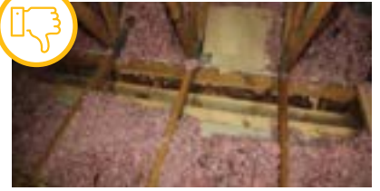
Open/unsealed chase or cavity. Courtesy of Oregon Housing and Community Services and Oregon Energy Coordinators Association
