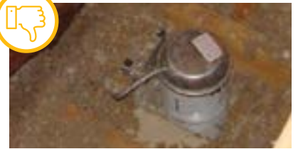
Unsealed non-IC fixture. Courtesy of Advanced Energy
