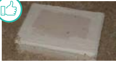
Non-IC fixture with drywall shield (hat). Courtesy of Advanced Energy
