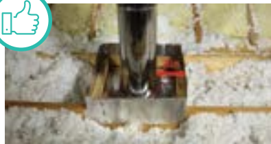
Non-IC fixture with drywall shield (hat). Courtesy of Advanced Energy
