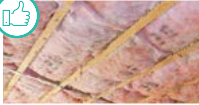
Insulation fills cavity, properly supported.
