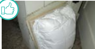
Crawl hatch insulated and weatherstripped.
