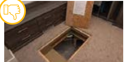
Crawl hatch NOT insulated or weatherstripped.
