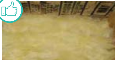
Insulation in full contact with floor.
