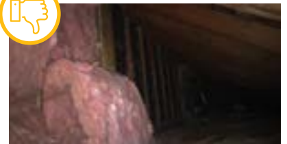
Open knee wall uninsulated. Courtesy of Advanced Energy
