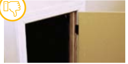
Uninsulated, not weatherstripped. Courtesy of Advanced Energy
