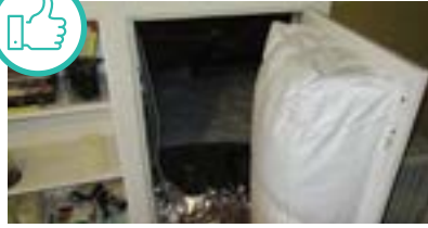
Weatherstripped and insulated hatch. Courtesy of Advanced Energy
