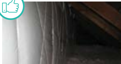
Open knee wall insulated and covered. Courtesy of Advanced Energy
