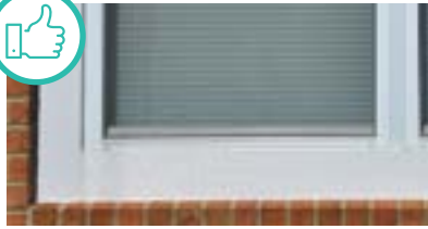
Double-paned window, installed with proper flashing.
