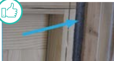
Backer rod and caulk complete seal around window frame. Courtesy of U.S. Department of Energy
