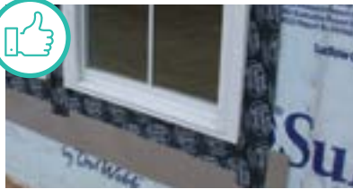
Proper flashing window to weather barrier. Courtesy of U.S. Department of Energy
