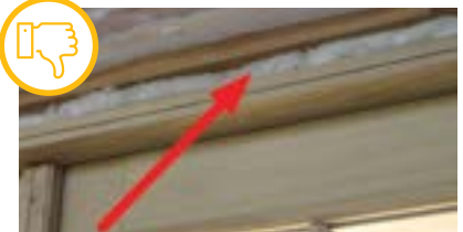
Incomplete seal around newly installed window. Courtesy of U.S. Department of Energy
