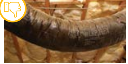
Duct is not properly supported.
