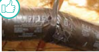
Duct properly supported.
