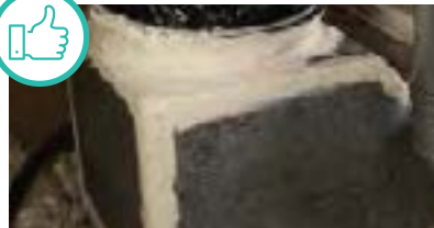
Plenum sealed with water based, fiber embedded duct sealing mastic.
