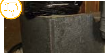
Unsealed duct plenum.
