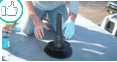
Roof penetration properly sealed. Courtesy of Oregon Housing and Community Services and Oregon Energy Coordinators Association
