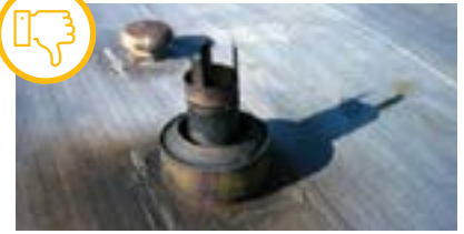
Penetrations should be sealed from the outside. Courtesy of Pennsylvania College of Technology
