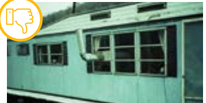
No skirting around home. Courtesy of Pennsylvania College of Technology
