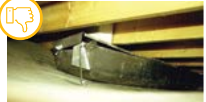
Uninsulated belly with duct leakage. Courtesy of Pennsylvania College of Technology
