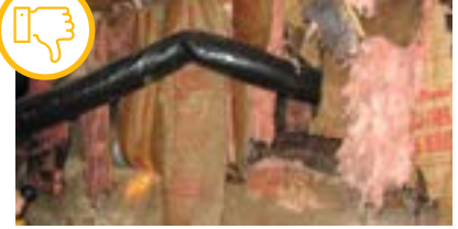
Unprepped crawl, disconnected dryer vent, poor ground cover. Courtesy of U.S. Department of Energy
