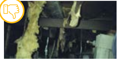
Belly is not whole. Courtesy of Pennsylvania College of Technology
