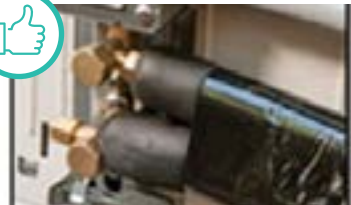
All line set/refrigerant lines properly insulated.
