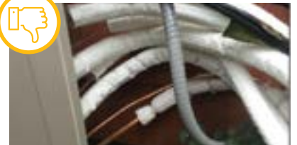
Line set/refrigerant lines not completely insulated.
